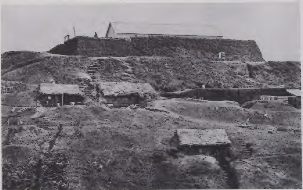
Fig. 22. Pahitere Redoubt from the east, showing dug-in soldiers’ huts, two with barrel chimneys, also a dovecote and well. A causeway over the outer ditch leads to the main entrance by way of a bridge across the inner ditch. Access to the ditch 5 m from the south-east corner gave a protected route into the redoubt from outside huts should the post come under attack, the main gate being very exposed. (Volume 2, Nicholl Album, Alexander Turnbull Library, Wellington).
